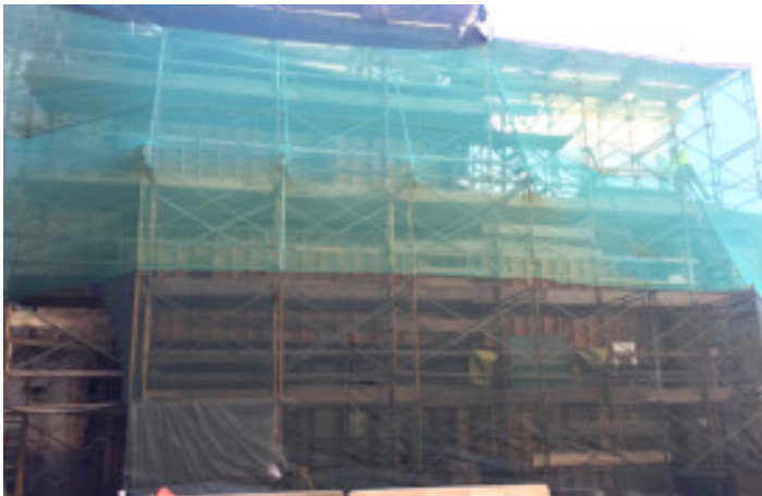
Figure 2. The scaffolding is braced by Jersey barricades enclosed with netting exposing completed demolition of brick walls and interior wood shoring walls.
