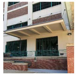
When all of the repairs were completed, Abbot painted the awning with an elastomeric paint to match the existing color and texture.
