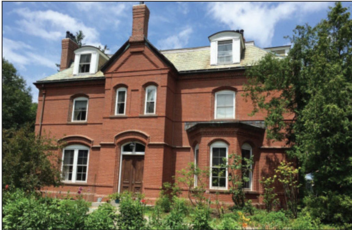
Victorian house in Milton, Mass: Abbot performed brick restoration on the north (left) side and west (front) sides of the house in separate phases. As evidenced by the photograph, the appearance of the brickwork is identical demonstrating the consistency and quality of the workmanship throughout the both phases.
