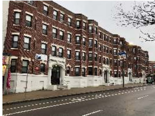
Figure 1. Blue Hill Ave. Apartments
