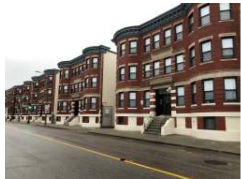
Figure 3. Washington St. Apartments
