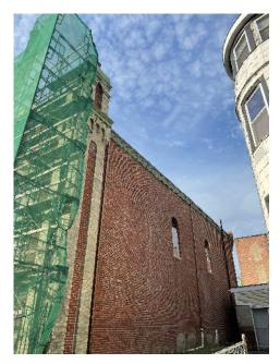
pipe staging to access the entire wall allowing a series of test holes to be created in areas specified by the architect. Based on this evaluation, it was determined that certain areas needed to be completely demolished and rebuilt with new brick to match the color and texture of the existing brick. The back-up wall also required repair as needed.
