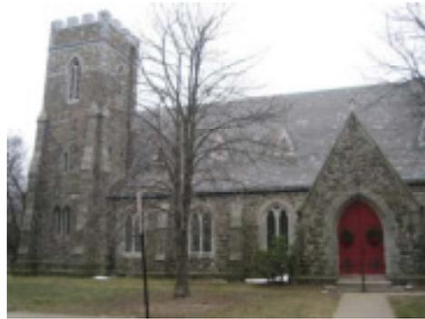
The original design of the church featured a 32-foot hexagonal stone steeple extending above a 52-foot rectangular stone and granite tower. In 2001, an engineering firm (Structures-North, Salem, MA) was contracted by the owner to evaluate the structural integrity of the steeple. The firm determined that the steeple was severely deteriorated and recommended that it be removed.
