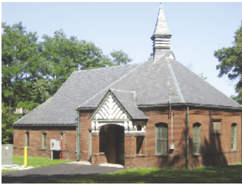
Hegarty Pump Station - Wellesley, MA
