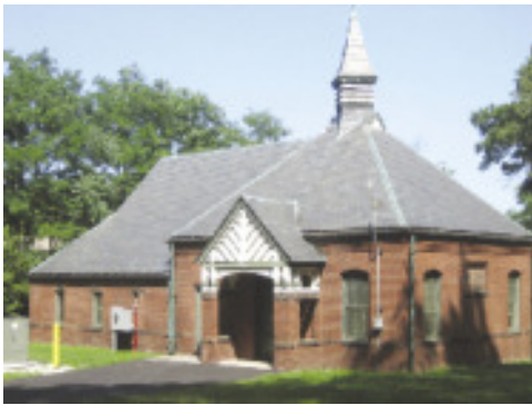
Hegarty Pump Station - Wellesley, MA
