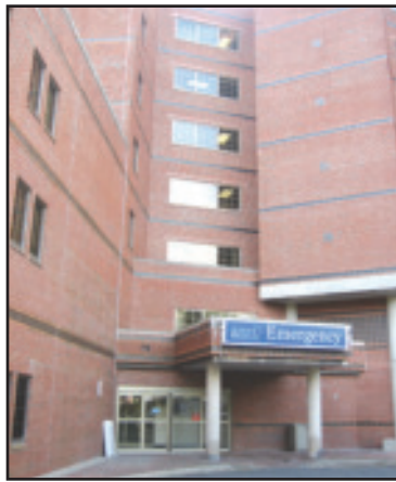
Emergency Room entrance, Quincy Medical Ctr., Quincy, Mass.
